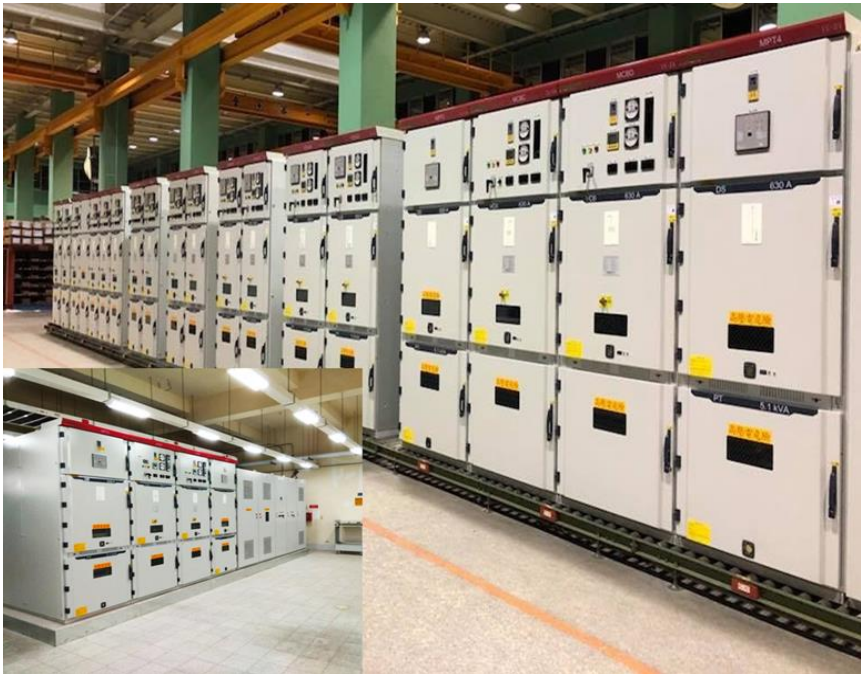
Taoyuan International Airport Terminal 2 Substation Replacement Project
