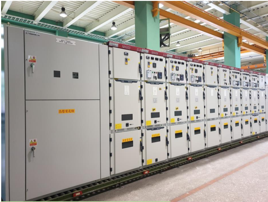
Ministry of transportation and communication new project of Tunnel Security Control
